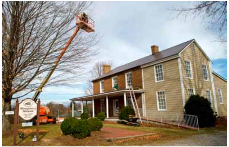
The museum roof was installed this fall.
