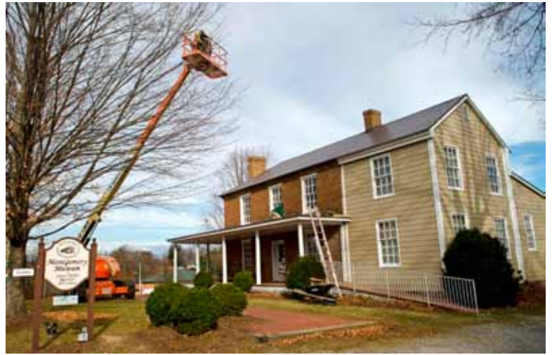
The museum roof was installed this fall.
